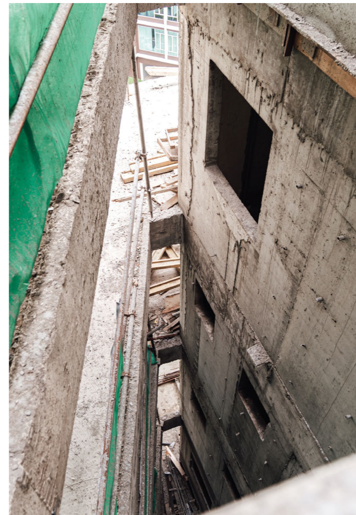
ATRIUMS: Voids separating the corridors from condo units. As a result, corridors are bright and airy, while offering residents privacy.
